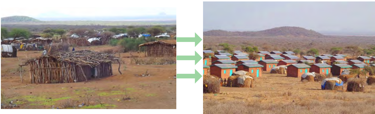
Fig- 19 Improved refugee shelters in Dillo and Megado camps, 2015
